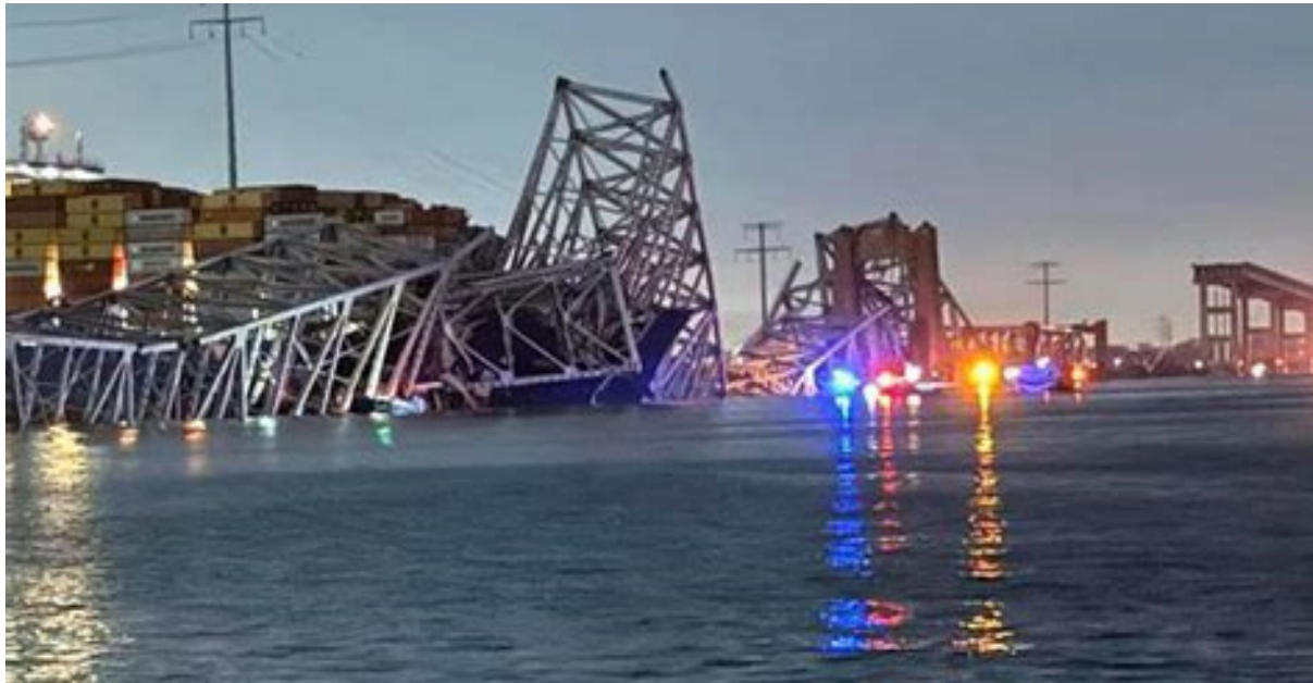
Collapsed Historical Baltimore bridge
